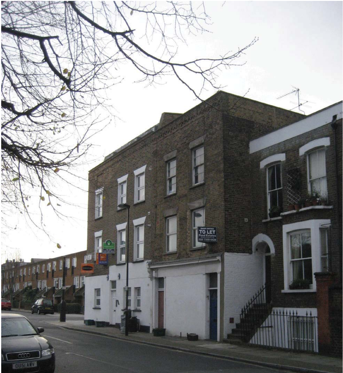
PROPERTY PRIOR TO DEVELOPMENT
